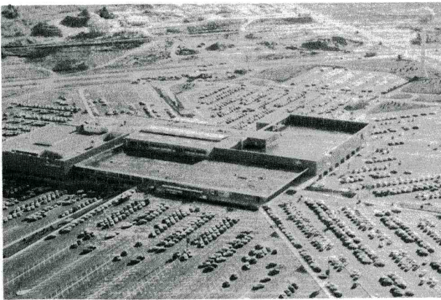
Soil-cement parking lot, Minneapolis, Minnesota. Room for 7000 cars.
